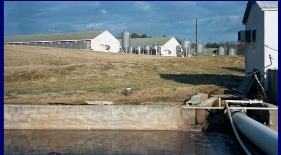
Hog CAFO including several confinement houses where the pigs are raised (background) and pipes leading from the buildings to the lagoon where the waste is collected (foreground)
