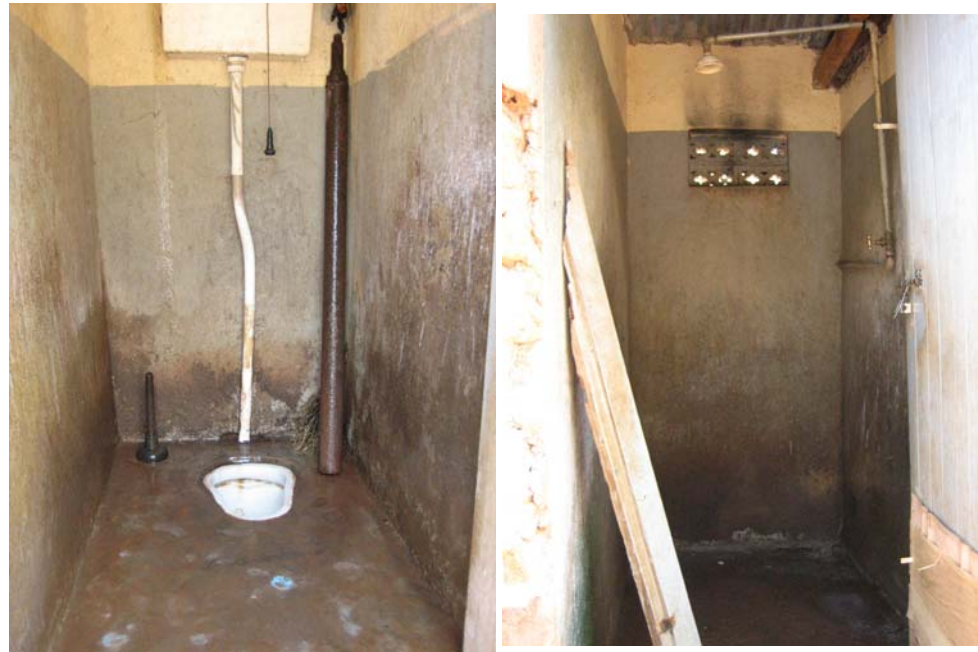
Toilet and shower in the nurse quarters yard
