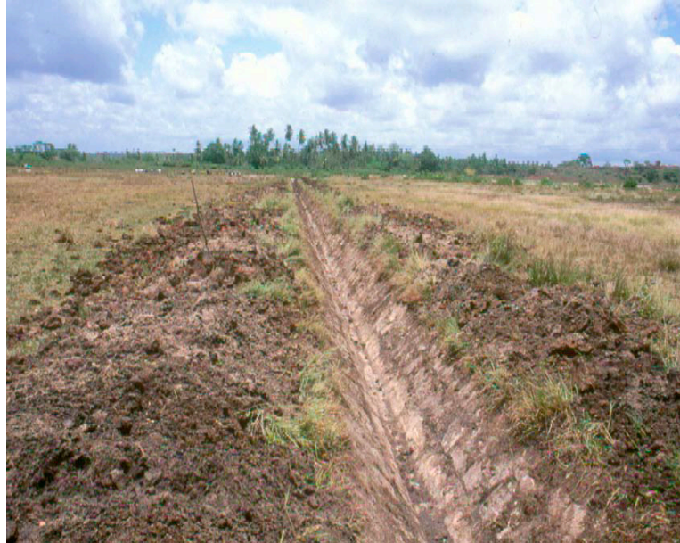
Successful Community Implemented Drain Rehabilitation Tanga, Tanzania
