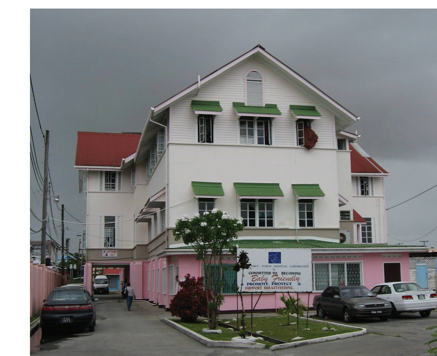
CECAP Center of Excellence and Training established at Georgetown Public Hospital.
