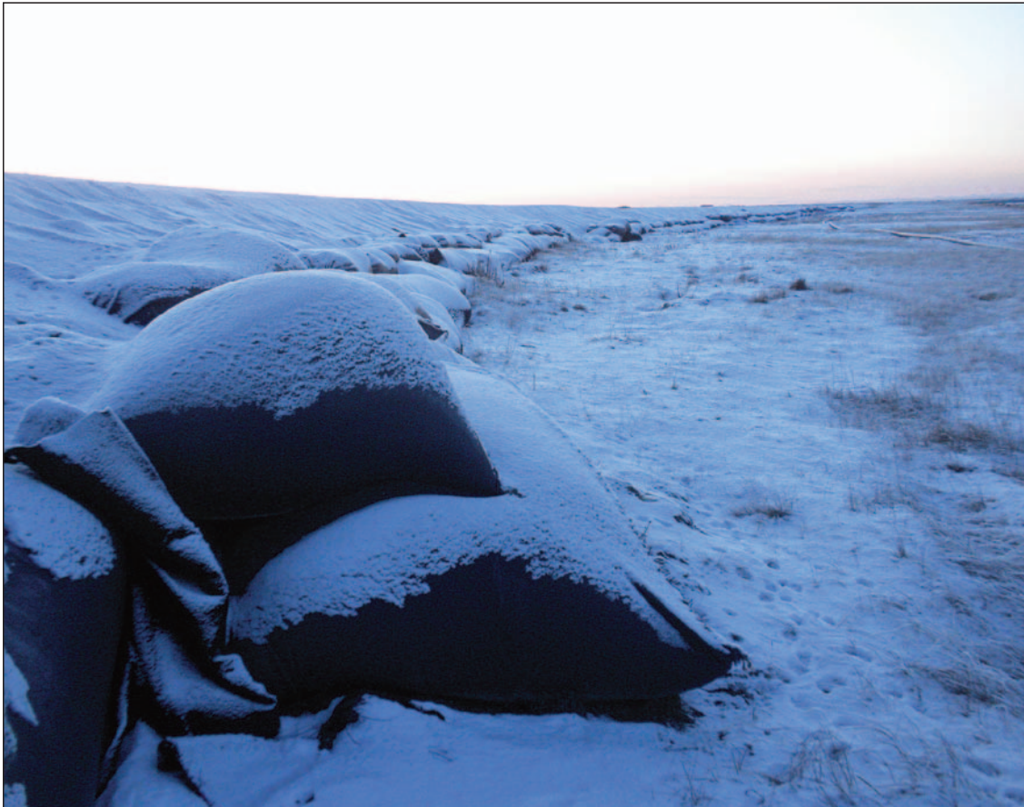
Evacuation road protection against erosion. Mike Brubaker 2009
