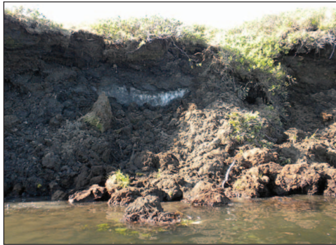
Rapid bank erosion occurring along the Kukpuk River.
