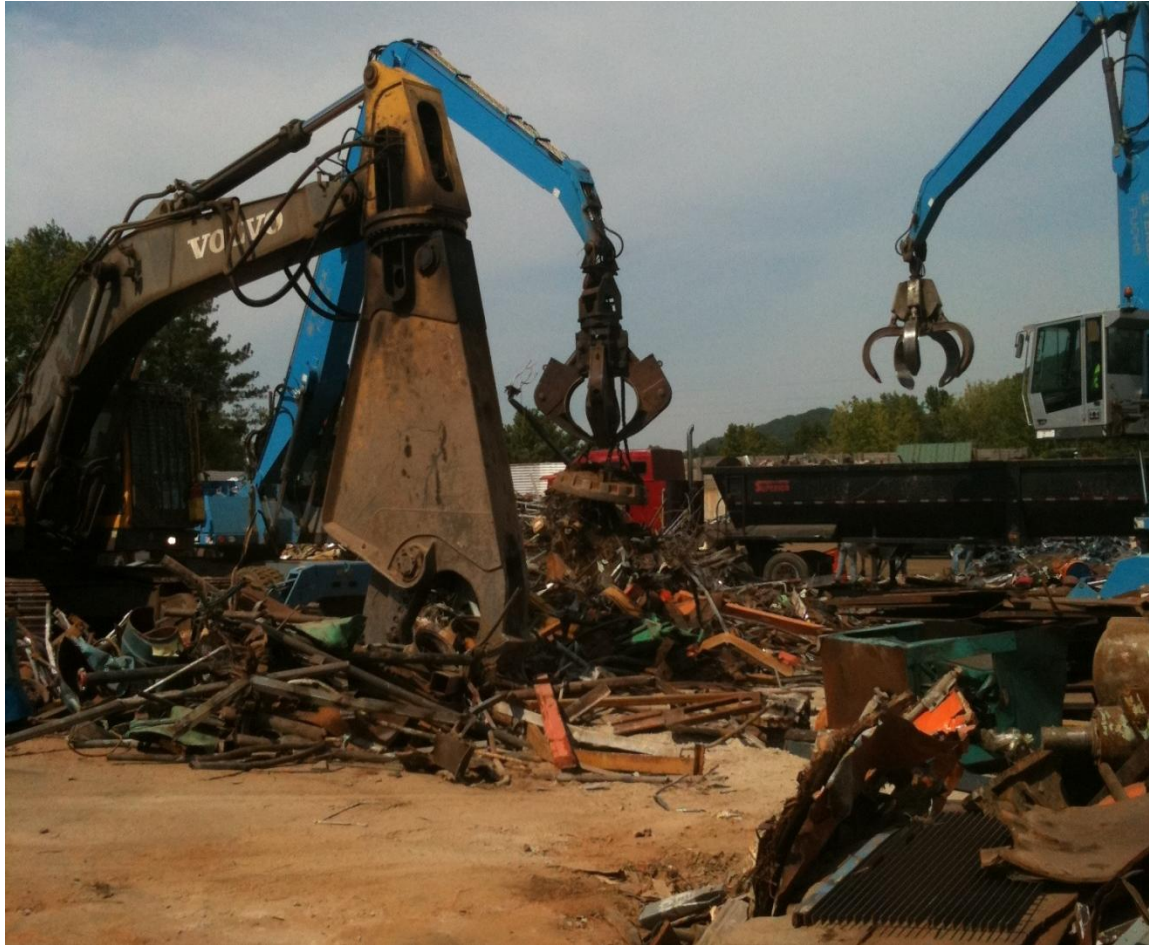
Mobile Hydraulic Shear Cutting (and Grapplers Staging Materials)
