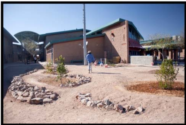
Lunch Space Renovation Challenger Middle School
