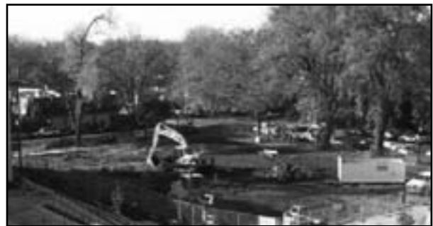
Construction underway at the Fremont Community Garden - Sacramento, CA
