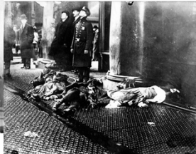
The fire at the Triangle Waist Company factory in New York City on March 25, 1911 killed 146 workers.
