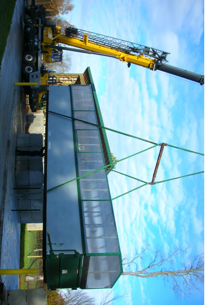
Above: a container based commercial composting system by Green Mountain Technologies being installed. Right: covered bays at a commercial composting facility.
