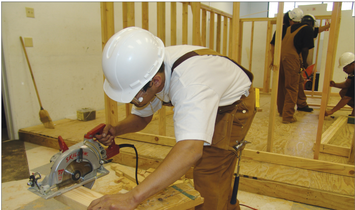
An OAI trainee cuts 2"x4" wood using the electrical Skilsaw.
