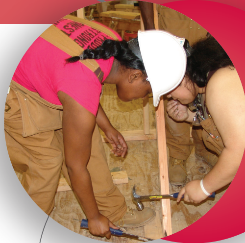
Two female CPWR trainees work together to erect a wall partition.
