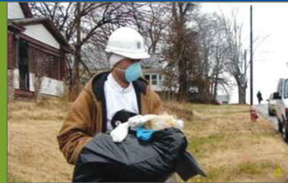
OAI trainee removes debris from vacant home.
